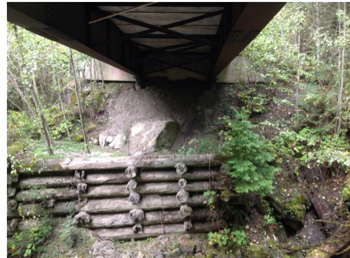
Right Bank Abutment when facing downstream
