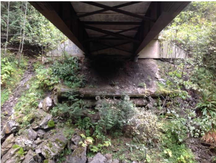
Left Bank Abutment when facing downstream
